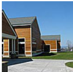
Check-Plus: Upstate Montessori School Earns Energy-Efficiency Honors
